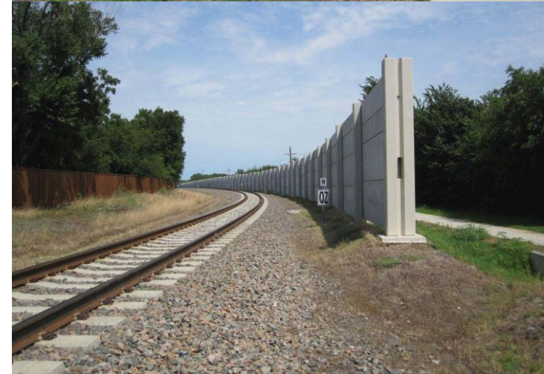
Example photos of noise barriers at rail projects.
