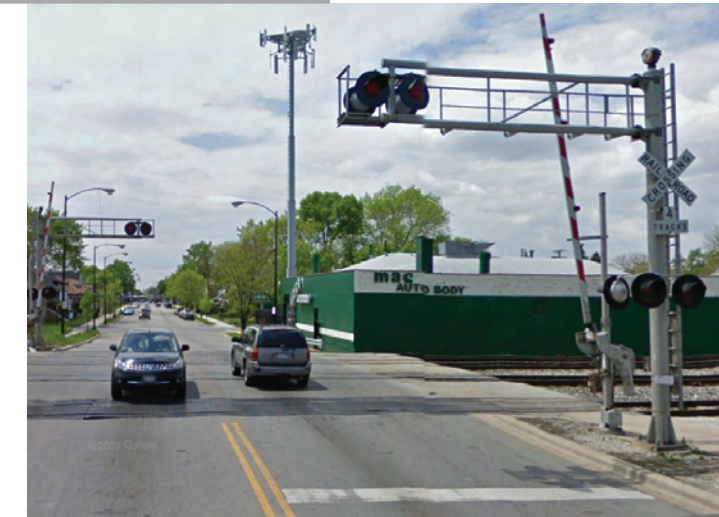
71st Street highway-rail grade crossing
