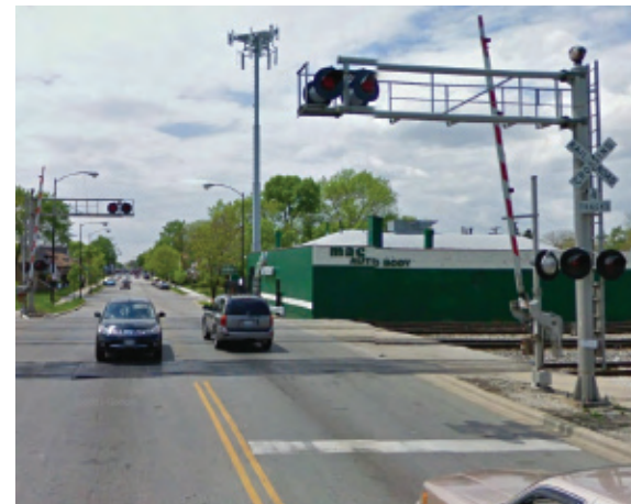
71st Street highway-rail grade crossing
