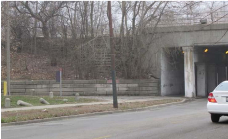
Figure 3.13-6: View of Area of Proposed Construction in Hamilton Park
