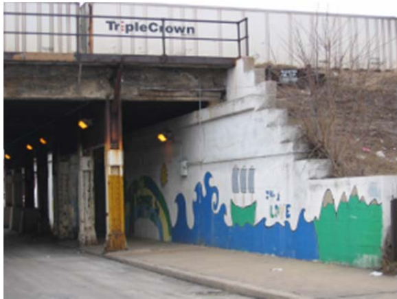
Figure 3.14-15: Morgan Street Bridge – East Abutment - Looking Northeast
