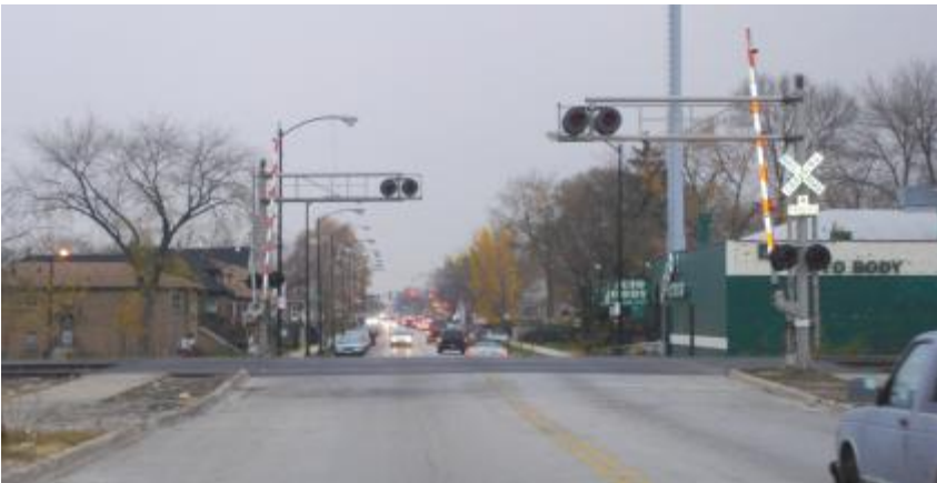
Figure 3.14-14: 71 st Street – looking west at CSX rail tracks
