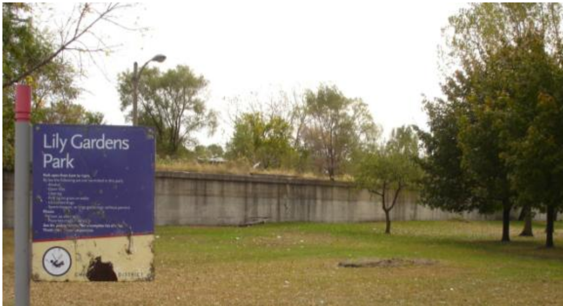
Figure 3.14-20: Railroad Embankment with concrete retaining wall in Lily Gardens Park
