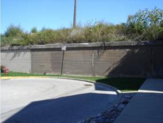
Figure 3.14-27: Example Retaining Wall at 400 W. 37 th Place
