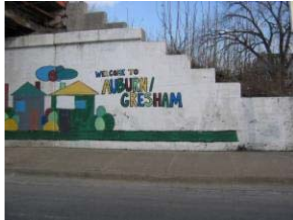
Figure 3.14-16: Halsted Street Bridge – East Abutment - Looking East
