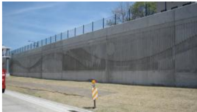
Figure 3.14-26: Concrete Retaining Walls along the Dan Ryan Expressway (I-94)
