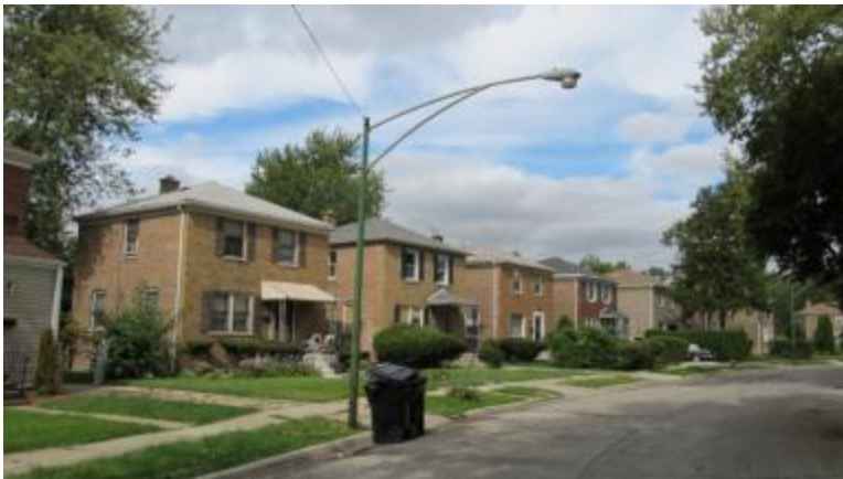
Figure 3.14-11: 7552 S. Hamilton Avenue – looking northwest
