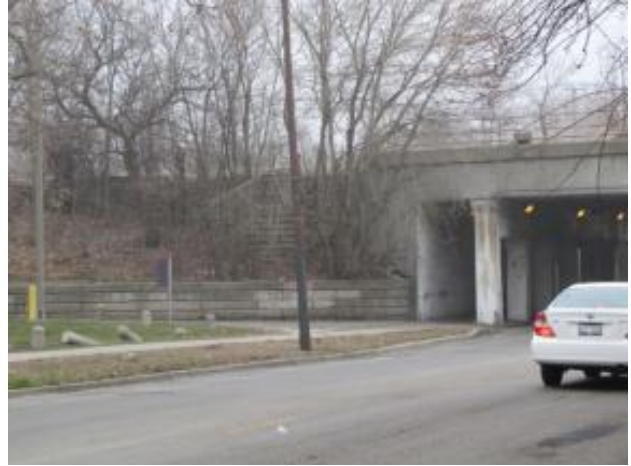
Figure 3.14-29: Retaining Wall to be Replaced in Southeast Corner of Hamilton Park
