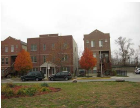
Figure 3.2-12: Residences on South Parnell Avenue near 76th Street
