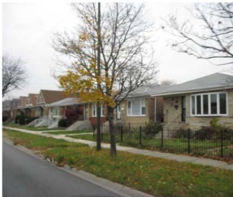
Figure 3.2-11: Chicago Bungalows located within the Study Area
