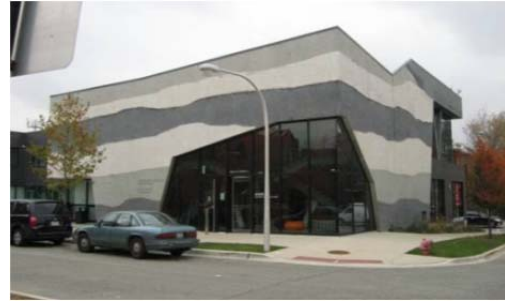
Figure 3.2-9: Lavezzorio Community Center, view from South Parnell Avenue
