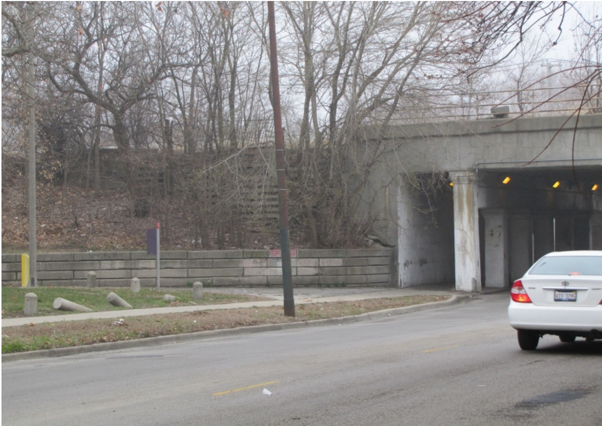
Figure 3.5-5: Hamilton Park and Existing Railroad Retaining Wall
