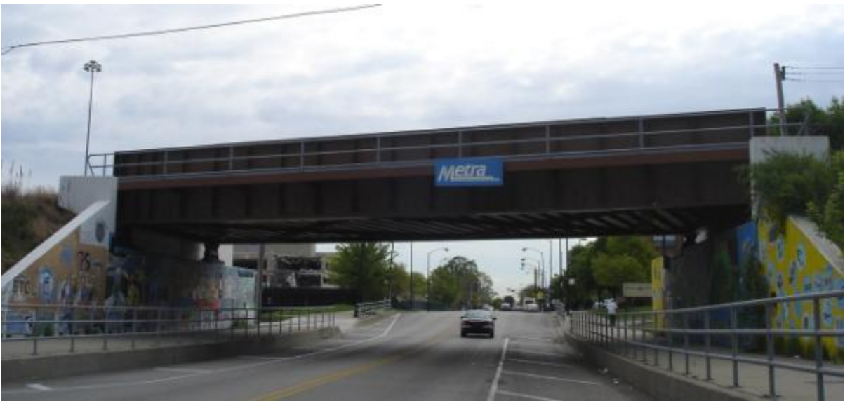
Figure 3.14-18: Newer railroad viaduct, Metra Rock Island District RR over 69 th Street
